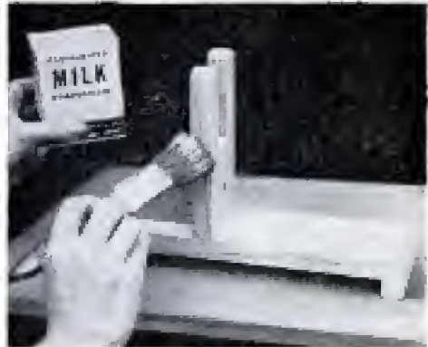
Above, there's no need to hunt for an empty can for small amounts of paint. A milk carton solves the problem nicely
